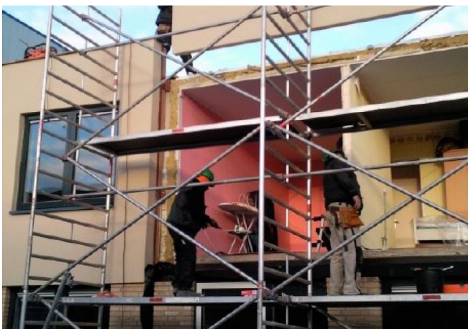
DURING THE PLACEMENT AND AFTER PLACING THE FACADE COMPONENTS [THINK WONEN, 2016]
