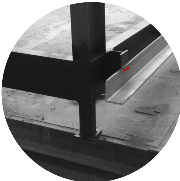
IN RED IS WHERE THE NEW BOLTED CONNECTION IS SITUATED.
