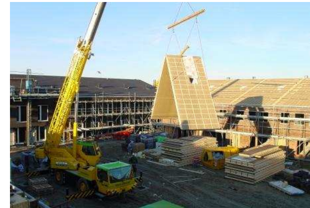
Fig. 39: Prefab methods speed up building process
